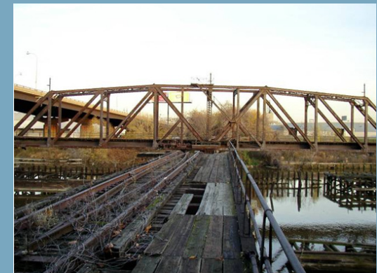
This railroad swing bridge was evaluated for its potential to serve as a pedestrian bridge across the Schuylkill River.
