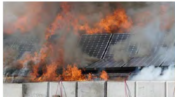
Figure 103 Roof and modules collapsing
