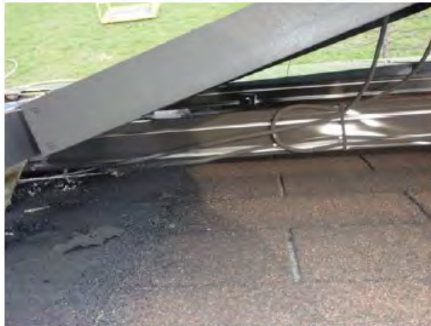
Figure 184 Looking under module for dangers
