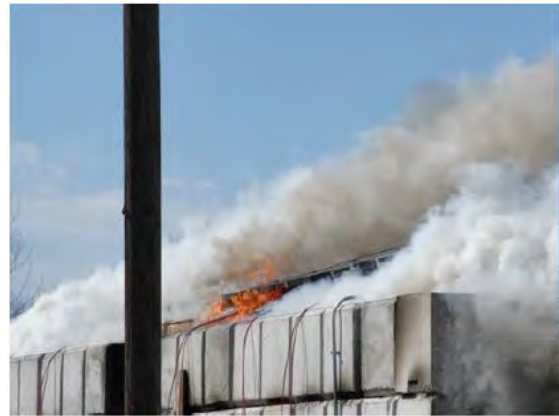
Figure 101 Open flames on roof
