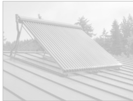
Solar Hot Water
