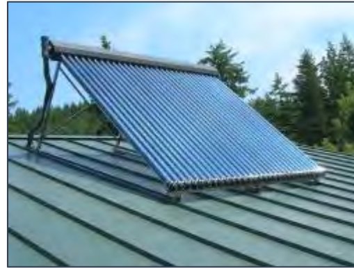
Solar Hot Water
