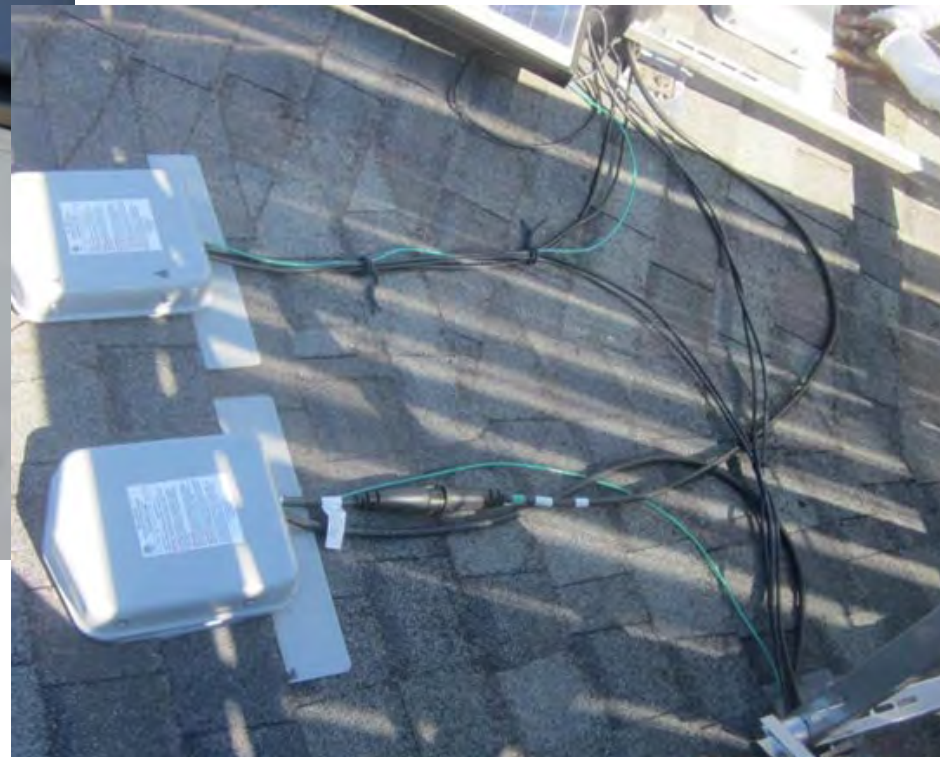
Poor wire management leads to additional hazards.
