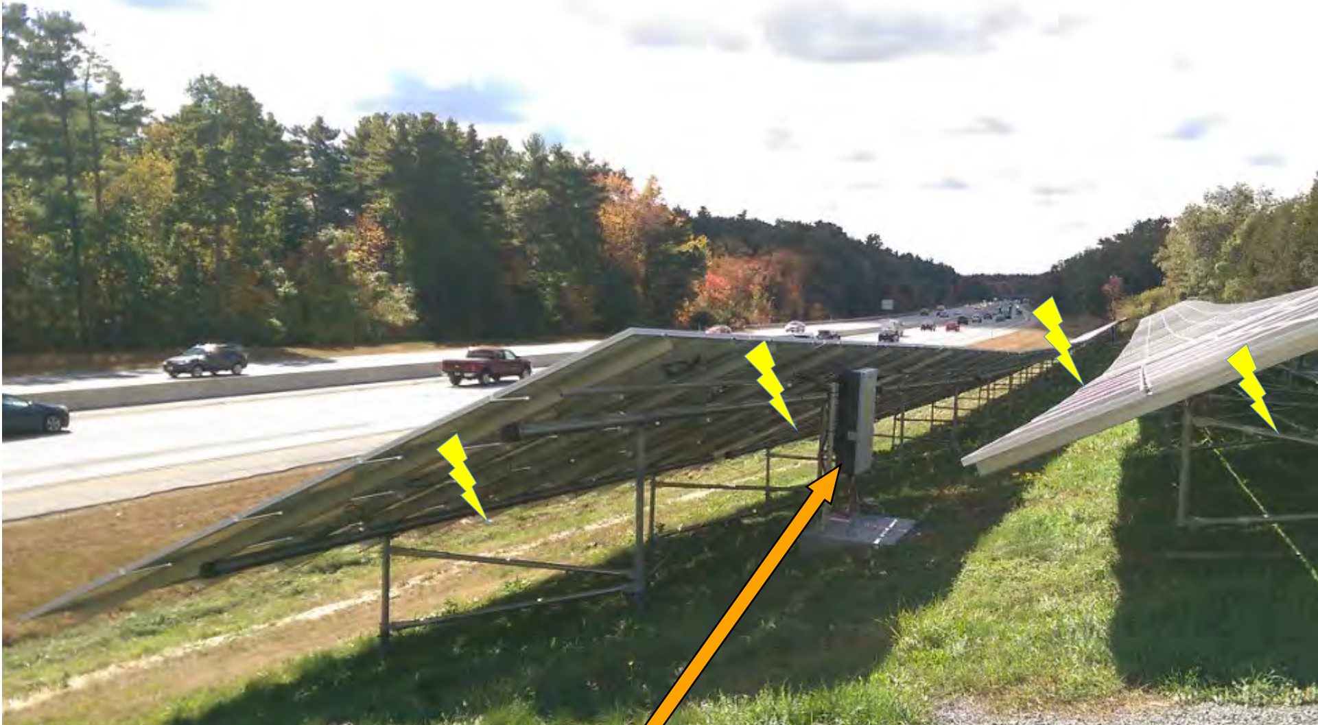
Location of inverter/disconnect. All other array conductors will remain energized when modules are exposed to light.
