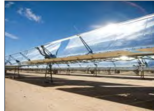
Concentrated Solar Power
