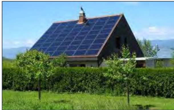
Solar Photovoltaic (PV)
