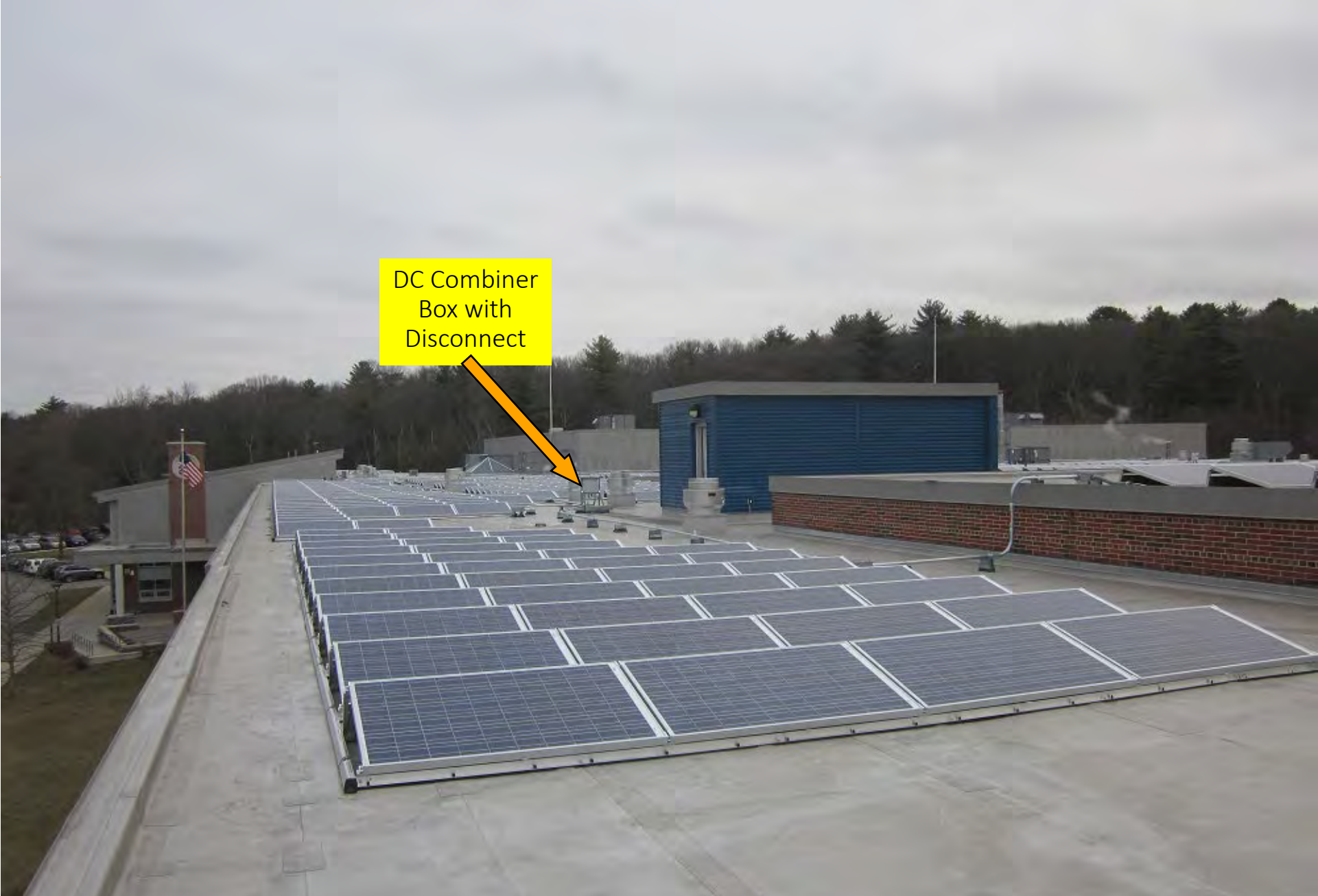
Example of commercial system. DC combiner contains disconnect, array will remain energized.
