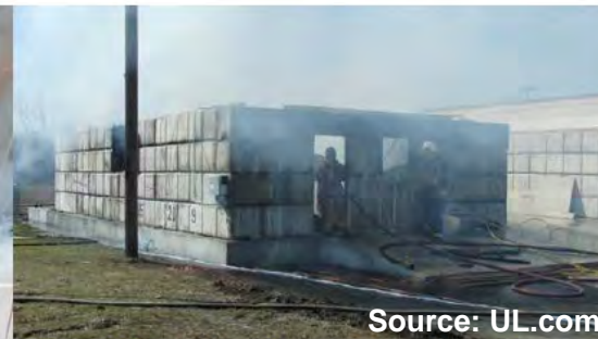
Figure 104 Roof collapsed -fire extinguished
