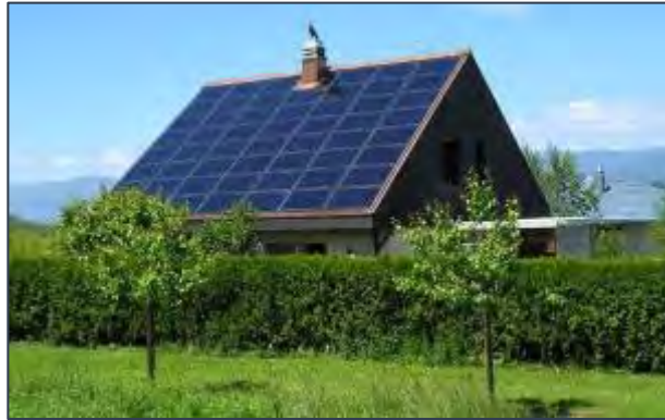
Solar Photovoltaic (PV)
