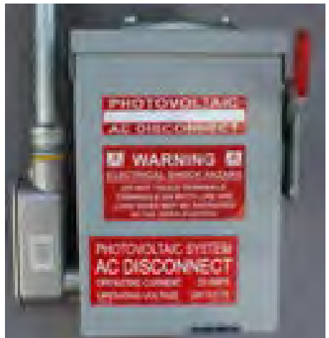
AC Disconnect Switch
