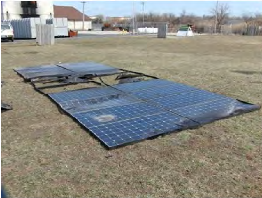
Figure 113 Post fire, front surface
