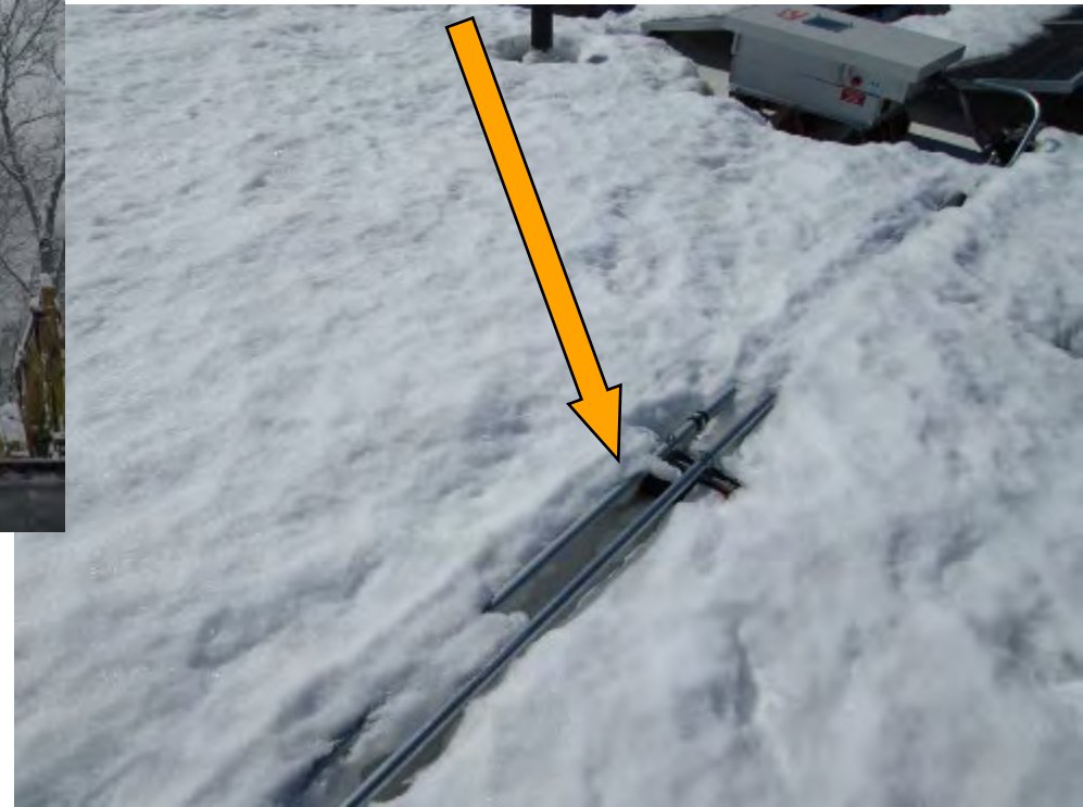
Rooftop conduits buried in snow.
