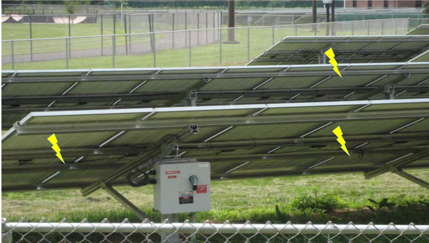
Ground-mount array with DC combiner/disconnect. Array conductors remain energized of disconnect is opened “off.”
