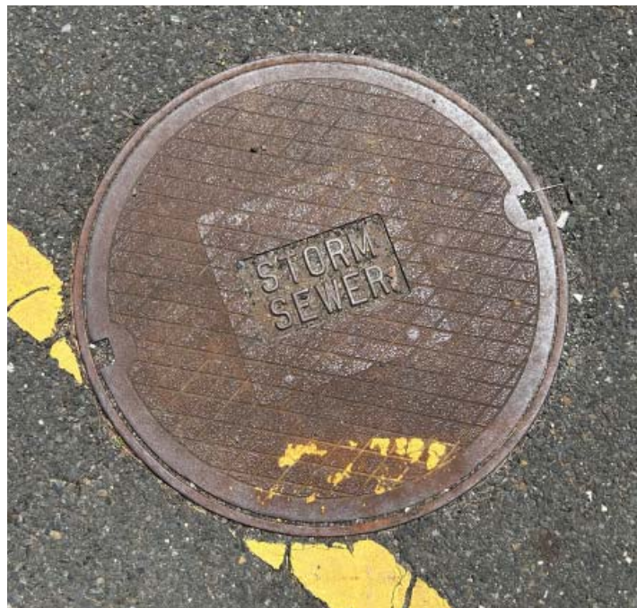
Storm Sewer in Hamilton Township
