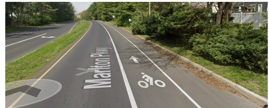
Figure 49: Existing Marlton Parkway bike lane
