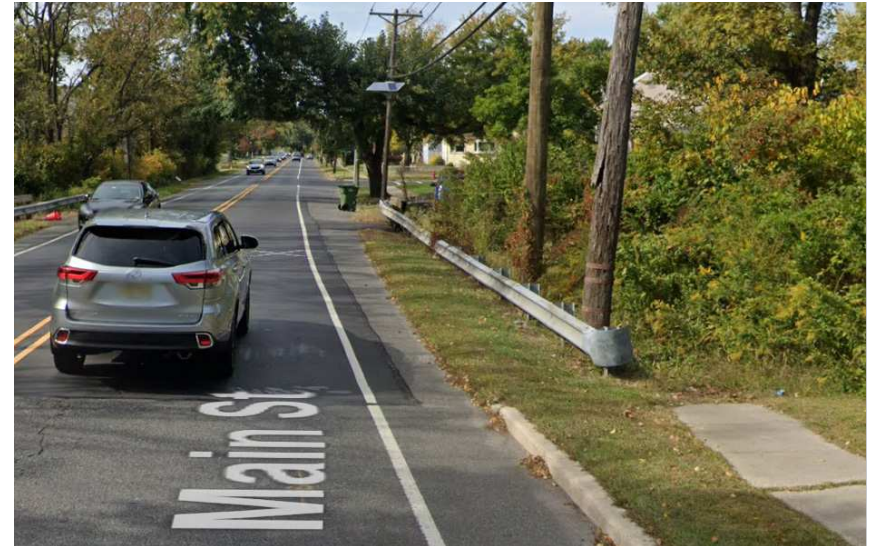
Figure 42: Sidewalk gap on Main Street east of Knox Road, Evesham, NJ, where a small bridge crosses a stream.
