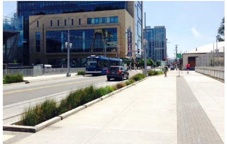
Bioswale in the curb zone, Portland, OR
