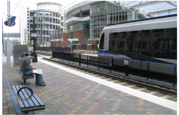
Transit Station, Charlotte NC
