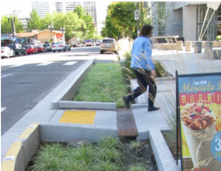
GSI curb extension
