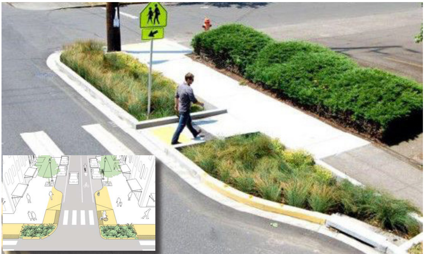
Figure 46 Curb extension with GSI
