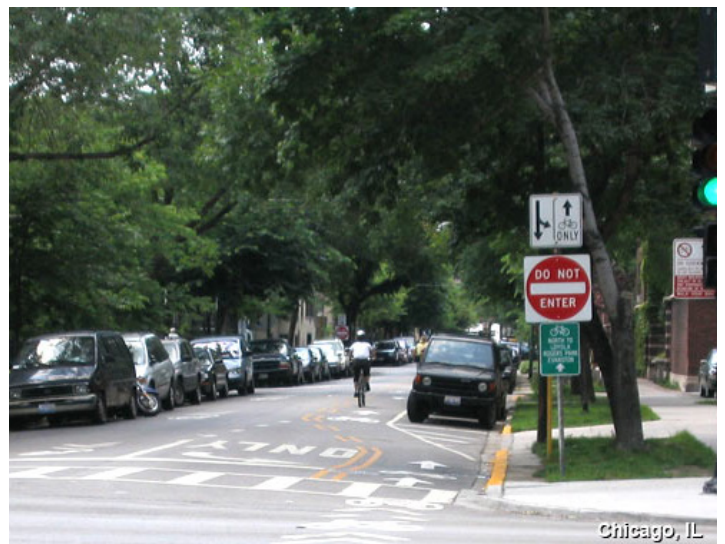
Contraflow bicycle lane, Chicago, IL
