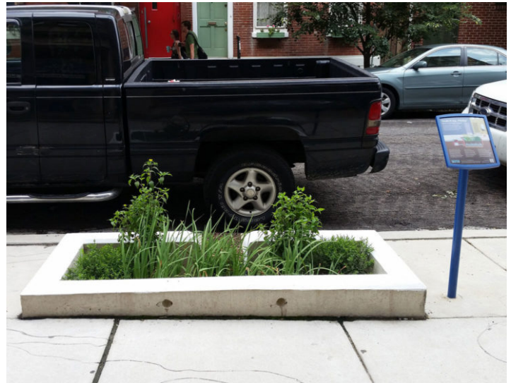
Small sidewalk rain garden in Philadelphia, PA
