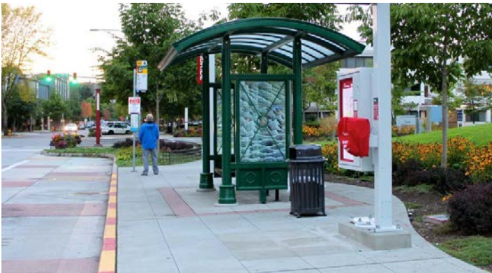
Bus shelter with amenities
