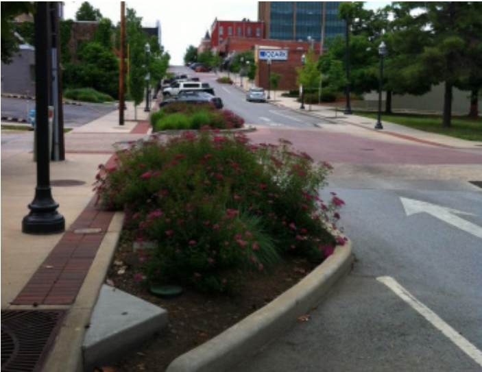
Green stormwater curb extension
