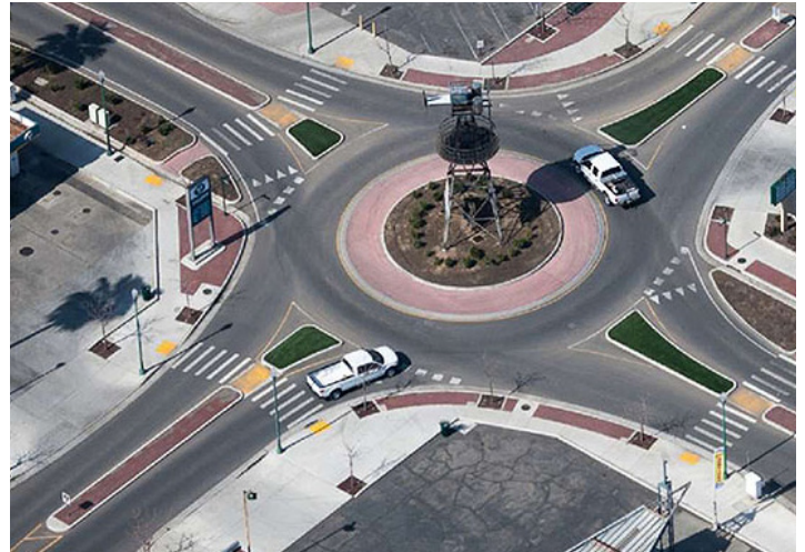
Roundabout with pedestrian islands
