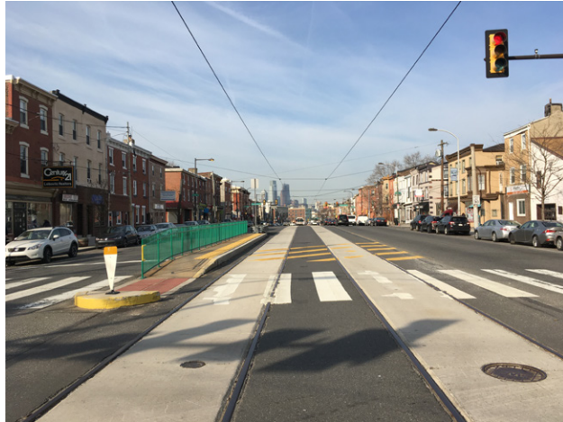
Figure 1: A typical existing Route 15 station
