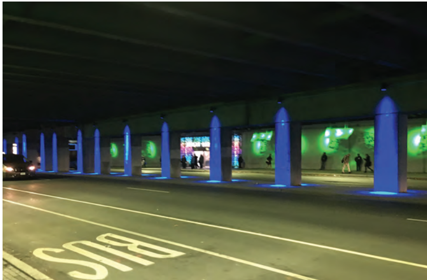
Underpass lighting at Spring Garden Station. Source: DVRPC, 2018
