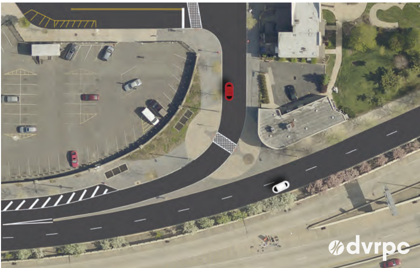
FIGURE 20: 9TH AND VINE WESTBOUND, EXISTING
