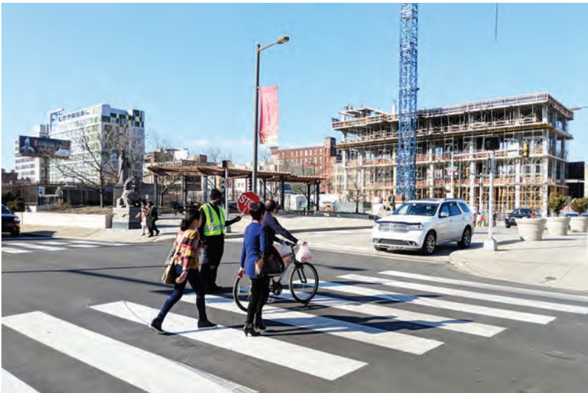
A crossing guard assists pedestrians crossing Vine Street eastbound at 10th Street. In the background, Eastern Tower is being constructed. Source: DVRPC, 2018
