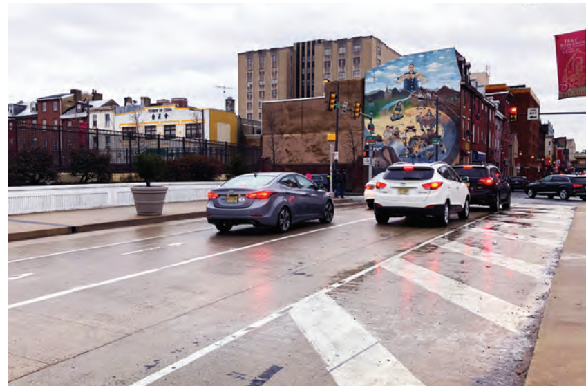
Vehicles frequently use the 10th Street bicycle lane due in part to low-visibility markings. Source: DVRPC, 2018
