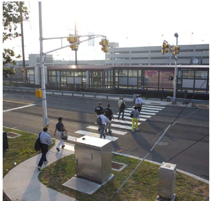
Pedestrian hybrid beacon provides improved pedestrian access across NJ 27 to Metropark rail station, where hundreds cross each day.
