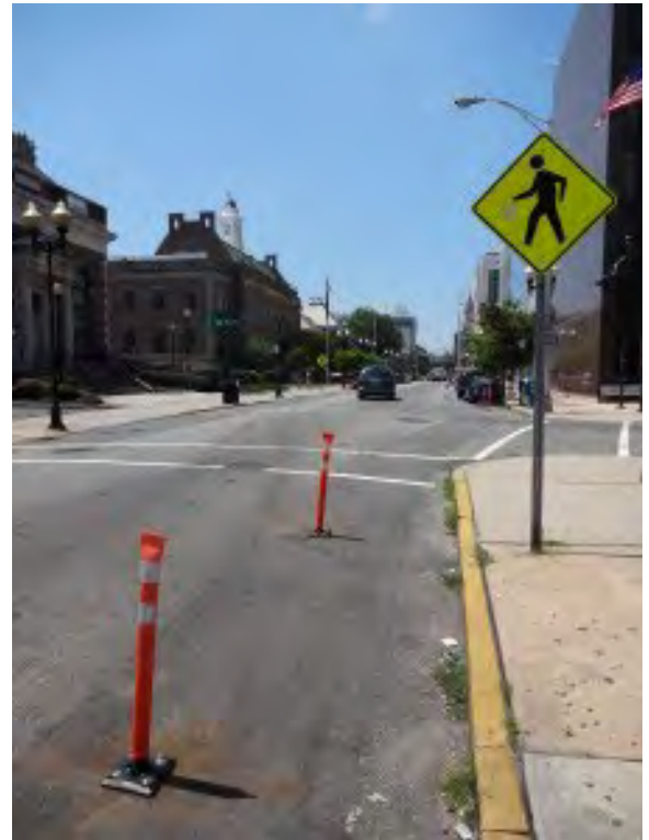
Daylighting on Bayard Street in New Brunswick, NJ
