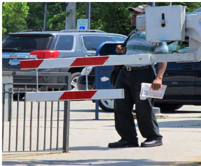
Pilot gate skirt improvements in Matawan, NJ aim to improve pedestrian safety at grade railroad crossings.
