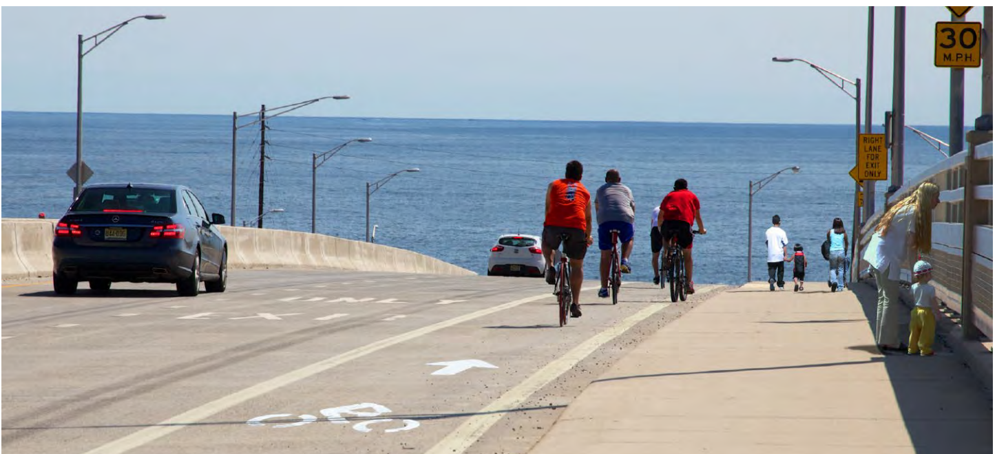
Bridge with bike lane in Highlands, NJ
