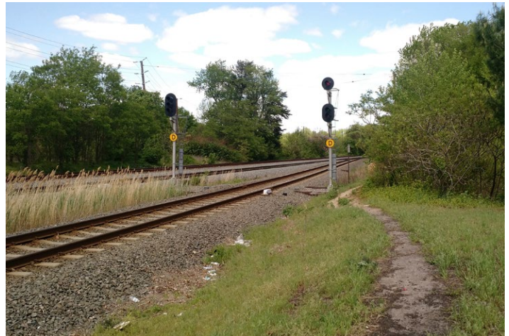
Recent employment growth has contributed to an increase in trespassing activity along the railroad right-of-way.
