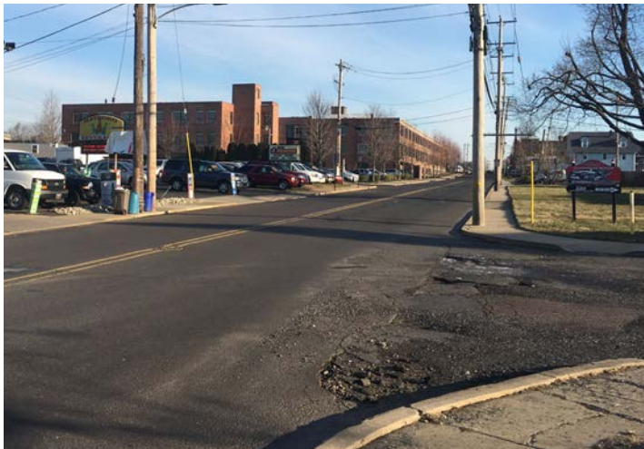
Jacksonville Road is scheduled for resurfacing in 2019.
