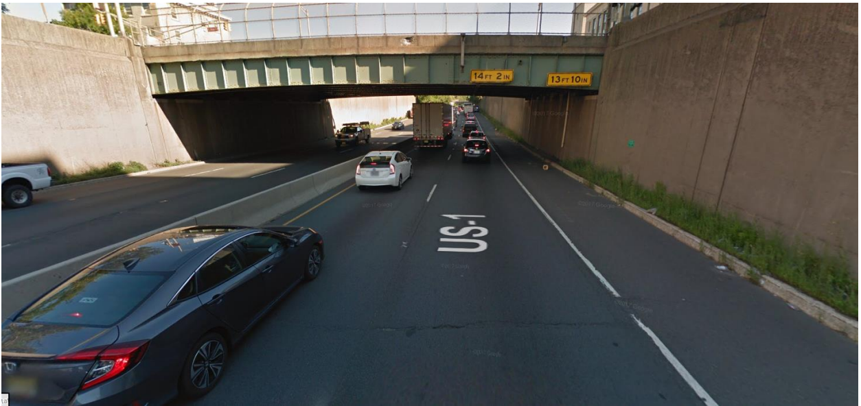
Figure 13: US 1 NB at State Street; traveling lane maximum height clearance 14' 2" and shoulder 13' 10". Source: Google Street View, October 2018
