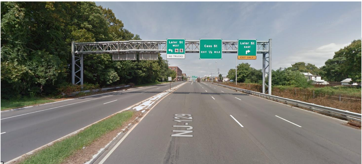
Figure 6: NJ 129 NB approach to CR 650 (Lalor Street); trucks prohibited from making left-turns. Source: Google Street View, October 2018
