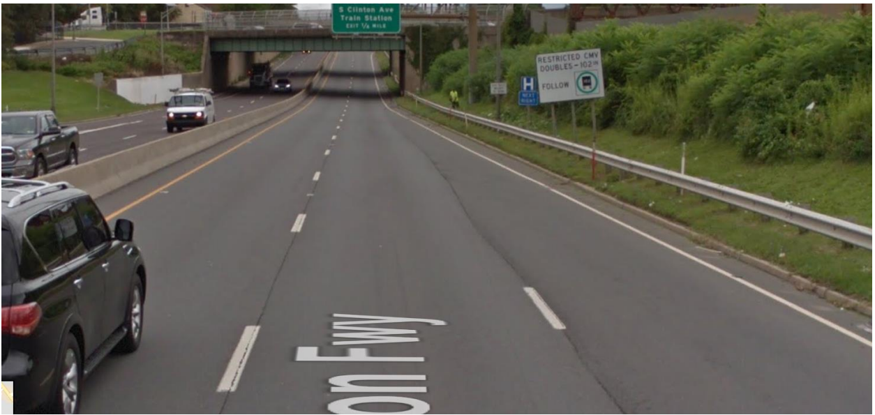
Figure 1: US 1 NB between NJ 29 and NJ 33 East exits; designated doubles 102" Commercial Motor Vehicle. Source: Google Street View, June 2018
