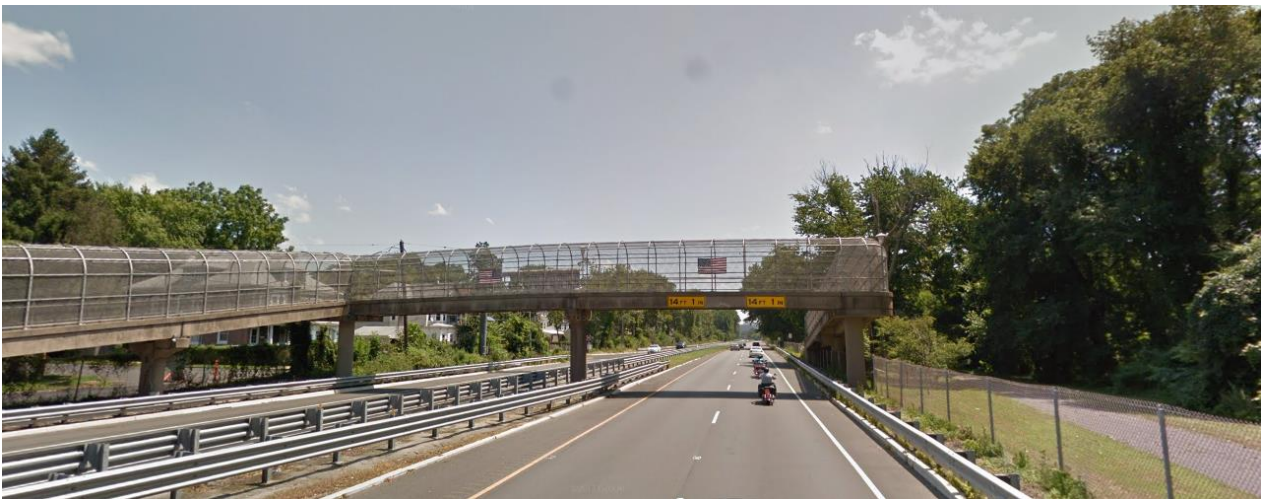
Figure 14: NJ 29 SB between Parkside Avenue and Morrisville, PA exit; maximum height clearance for pedestrian bridge (14' 1"). Source: Google Street View, October 2018
