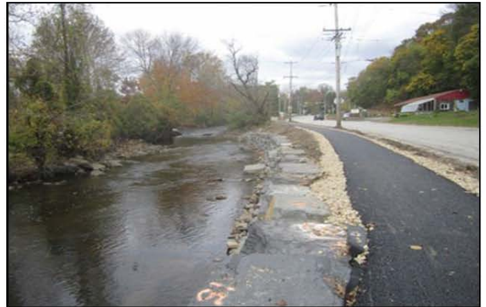
Recent Transportation Enhancement dollars provided for new stream bank stabilization. Also shown is the new pedestrian/bicycle trail. Source: DVRPC.
