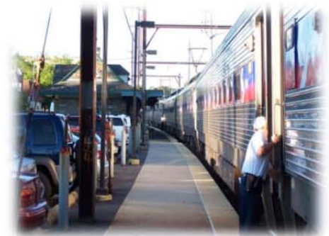
Shown above is the existing Willow Grove station platform. The feasibility study examined improved safety and station access for commuters.
