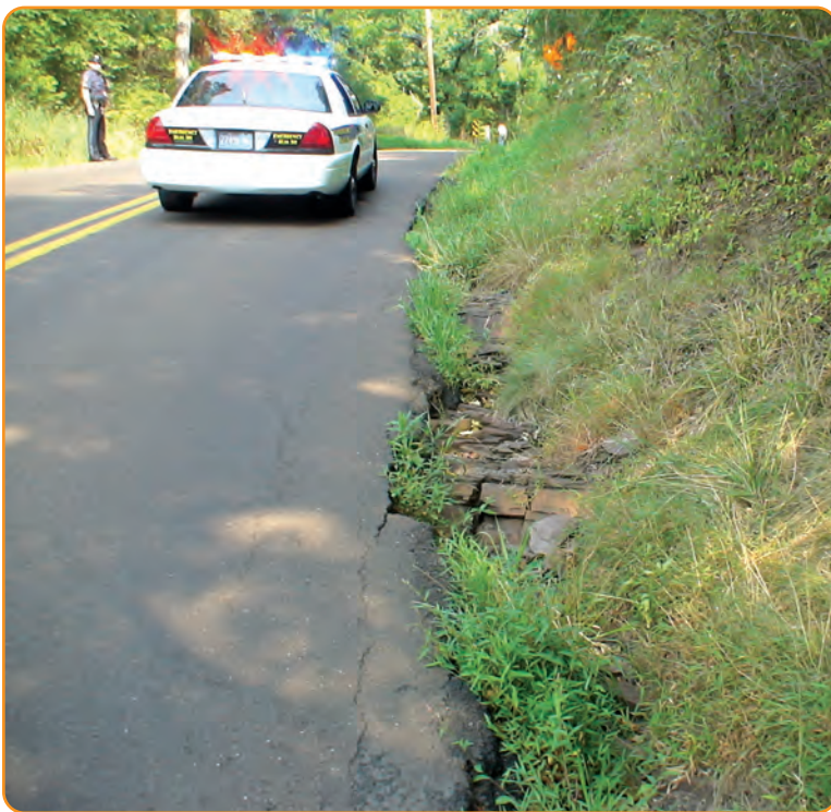
Improving safety involves engineering, enforcement, education, emergency services, and policies.
