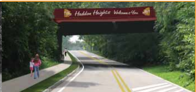
AFTER: SIDEWALKS, RESTRIPING OF THE ROADWAY, SPEED LIMIT PAVEMENT MARKINGS, RUMBLE STRIPS, AND MORE SIGNAGE WOULD SLOW TRAFFIC AND INCREASE SAFETY FOR PEDESTRIANS
