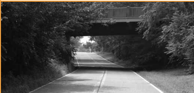
BEFORE: EXISTING CONDITIONS ON ATLANTIC AVENUE NEAR HADDON HEIGHTS ELEMENTARY SCHOOL
