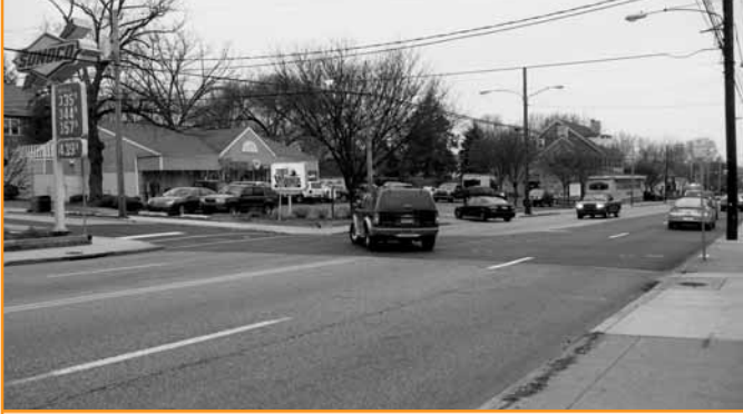
BEFORE: EXISTING CONDITIONS ON BETHLEHEM PIKE NEAR THE INTERSECTION WITH MILL ROAD
