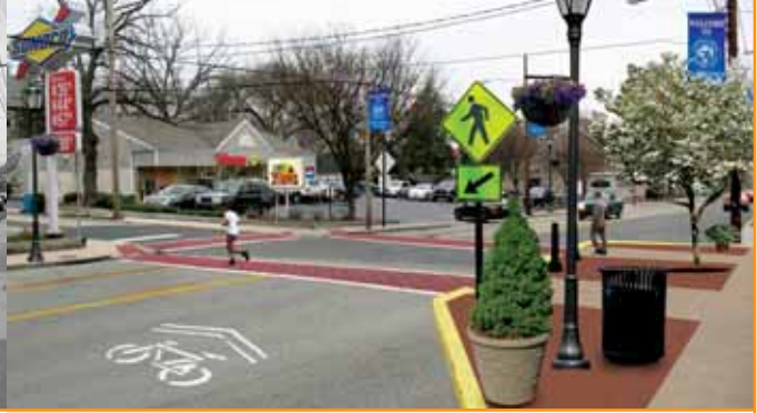
AFTER: PHOTO SIMULATION OF RECOMMENDED IMPROVEMENTS SHOWS A NEW CROSSWALK, A THREE-LANE CROSS-SECTION, SHARED-LANE MARKINGS, A DEDICATED PARKING LANE, STREETSCAPING, AND CURB EXTENSION
