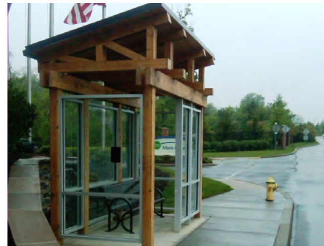
Figure 30: Custom Shelter in Glen Mills, PA
