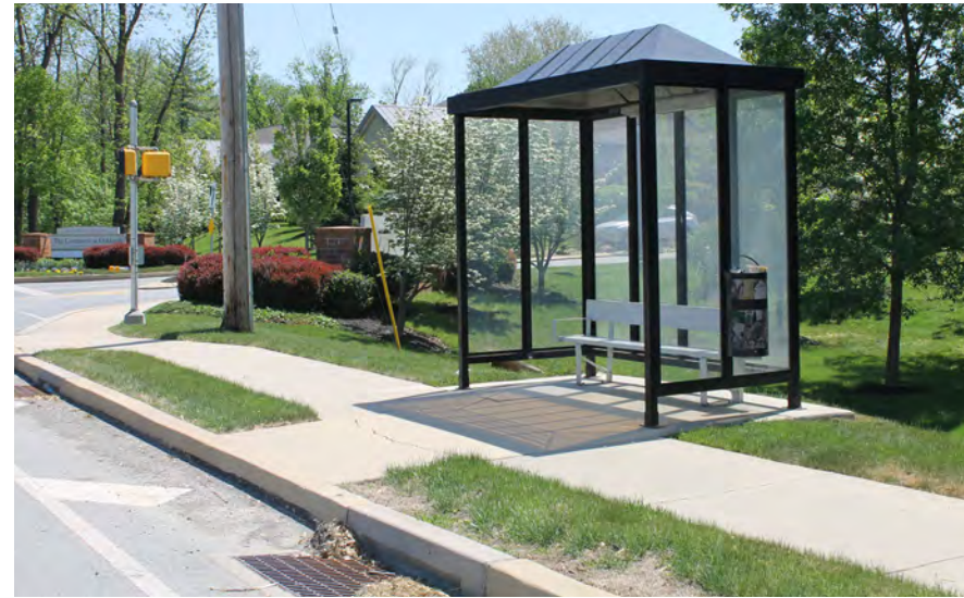
Figure 19: Waiting Area with Standard Shelter
