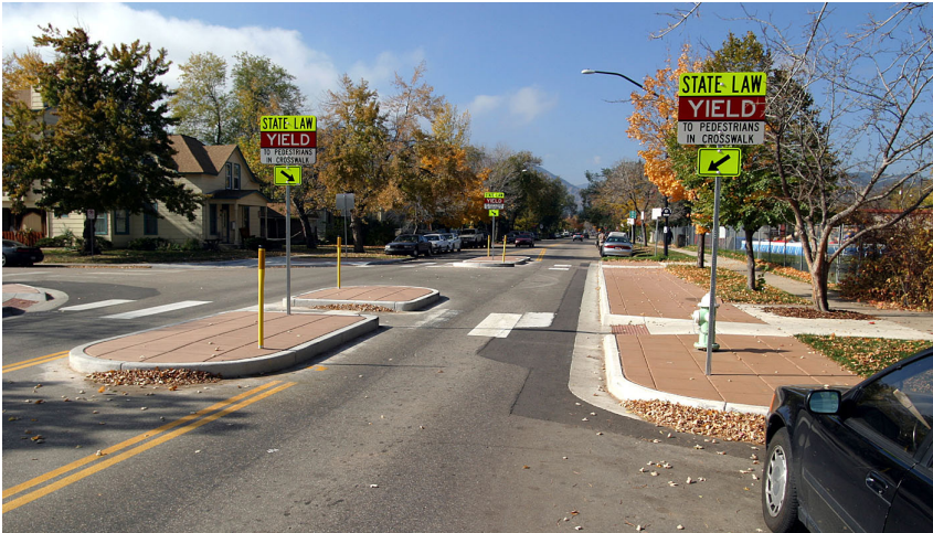
Figure 4: Pedestrian Refuge Island and Curb Extension
