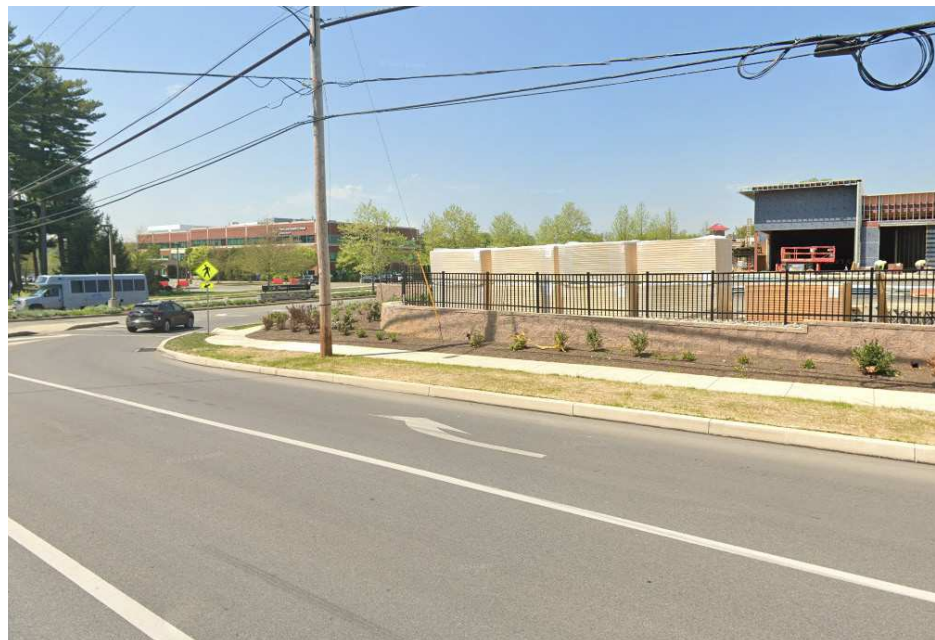
Figure 18: Sidewalk Facilities at Large Development Site
