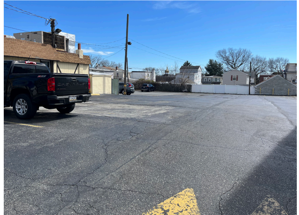
Figure 8: Underutilized Parking Lot
