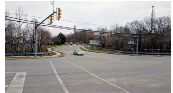
Even when sidewalks are present, large intersections with minimal crosswalks can make walking uncomfortable in some station areas.
