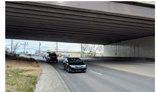
Narrow sidewalks next to high-volume roads contribute to an unpleasant pedestrian environment.
