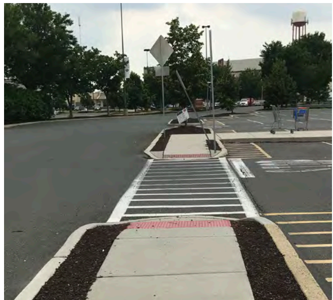
Figure 22 | Existing Pedestrian Facilities on Pier 70 Boulevard with Access to Walmart
