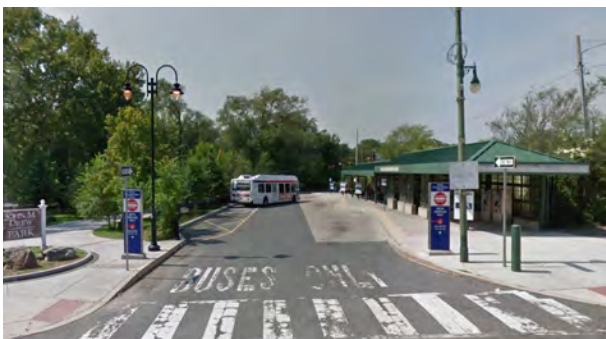
Figure 16 | Photos of Darby Transportation Center
