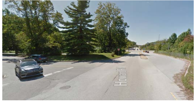
US 30 eastbound on-ramp where it meets Howard Road and Walkertown Road Source: Google (2016)
