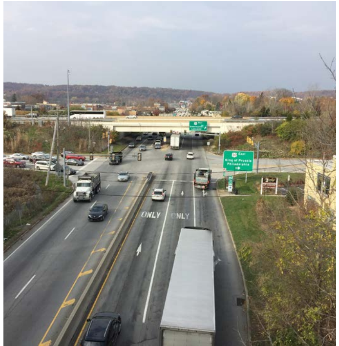
Major infrastructure Crossing of US 30 and PA-100 Source: DVRPC (2016)
