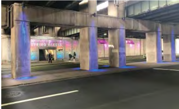
Figure 16: Spring Garden Street MFL Underpass
