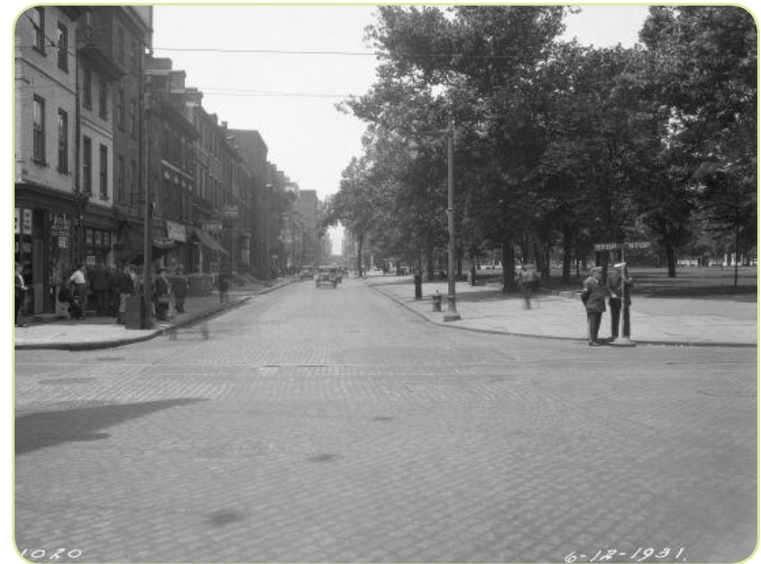
FIGURE 02: Original Street Configuration in 1931, Race and 6th Street looking west
