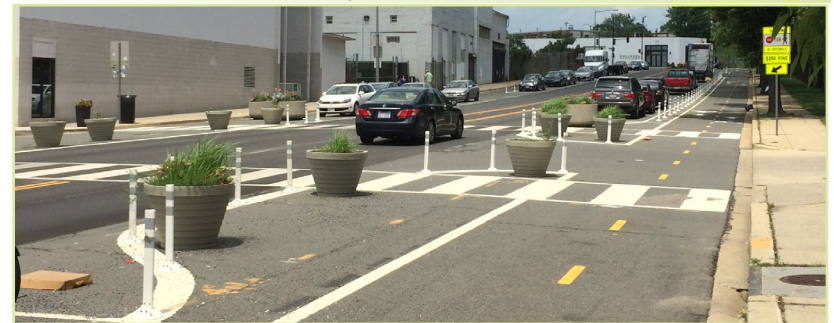
FIGURE 34: Example of Temporary Materials used to create a Curbside Protected Bicycle Lane with Pedestrian Areas
