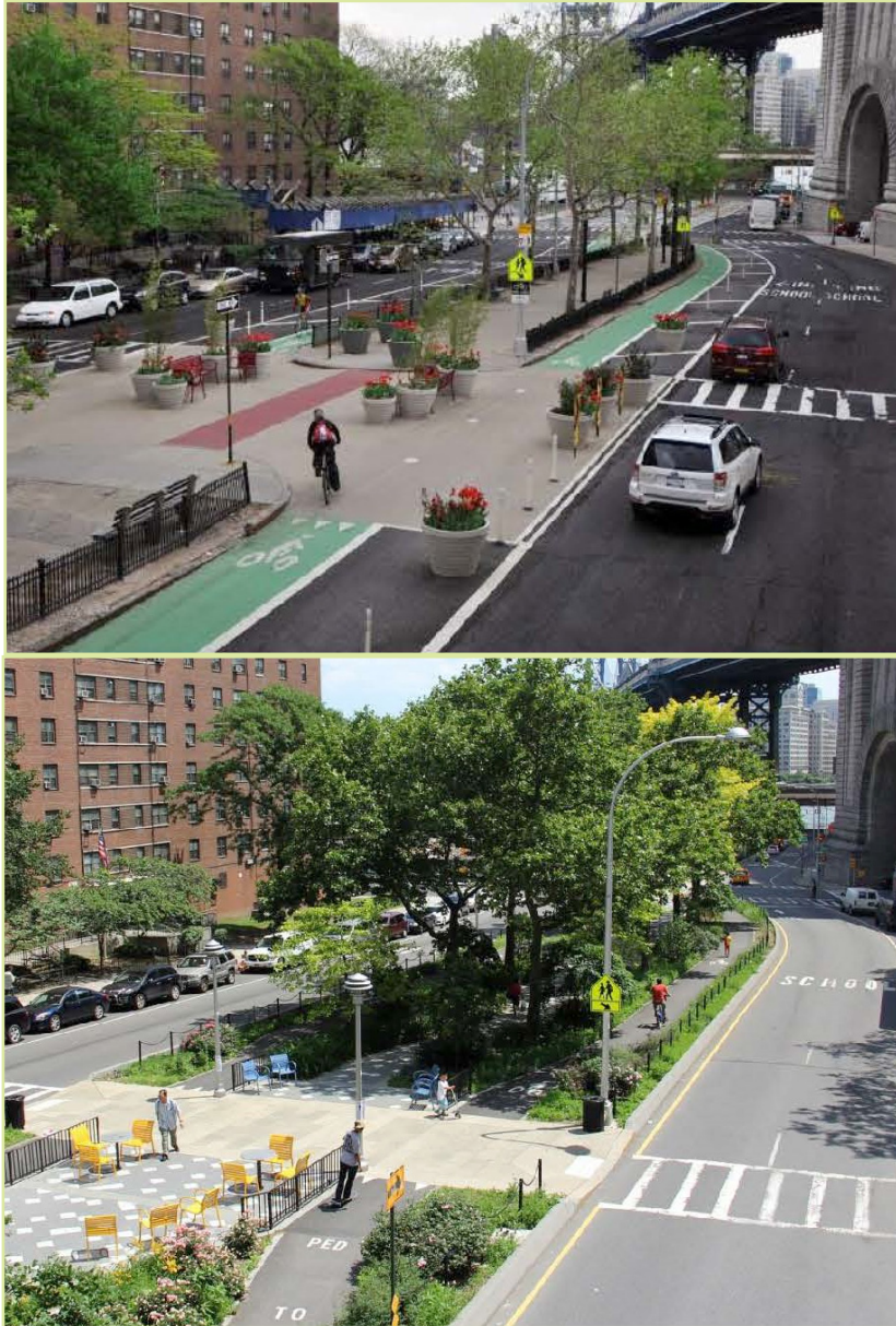
FIGURE 33: Example of Two-Stage Implementation with Temporary and then Capital Materials– NYC Department of Transportation Allen and Pike Street Improvement Project
