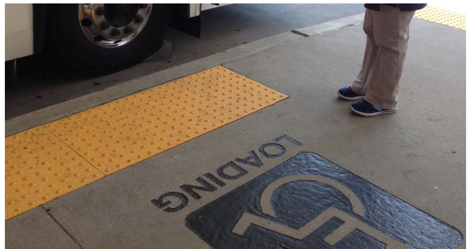
Figure 25: Landing Pad at SEPTA Bus Loop
