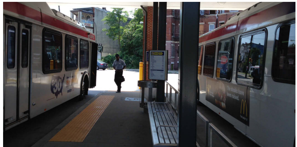
Figure 23: SEPTA Bus Waiting Area at 33rd and Dauphin Loop
