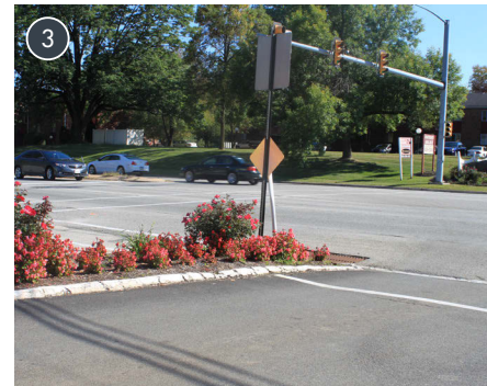
The crosswalk at Mary Fran Drive is interrupted by a landscaped median, potentially forcing pedestrians into the street.
