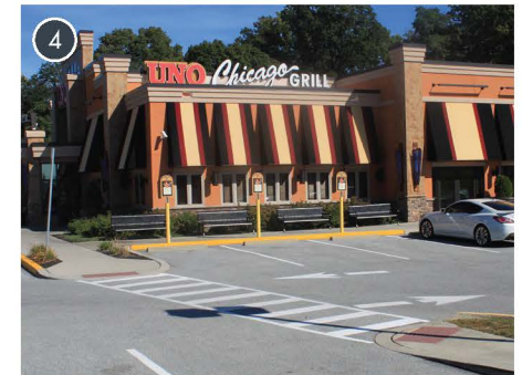
A system of internal sidewalks and crosswalks help walkers safely access the commercial development south of West Chester Pike.
