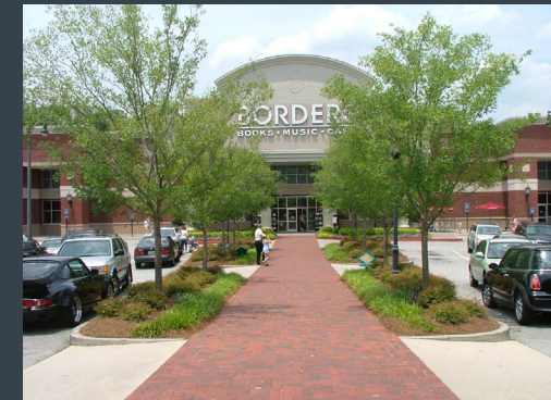
This shopping center uses a combination of speed tables and brick paving to create a high-visibility pedestrian route through the parking lot.
