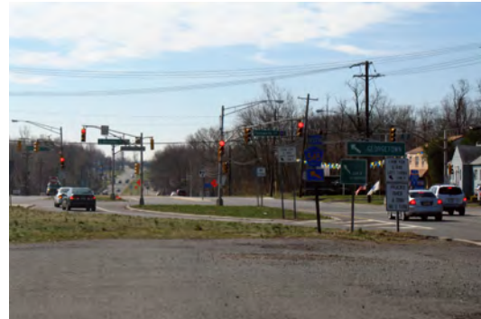
Ground-level view of the southbound left-turn lane
