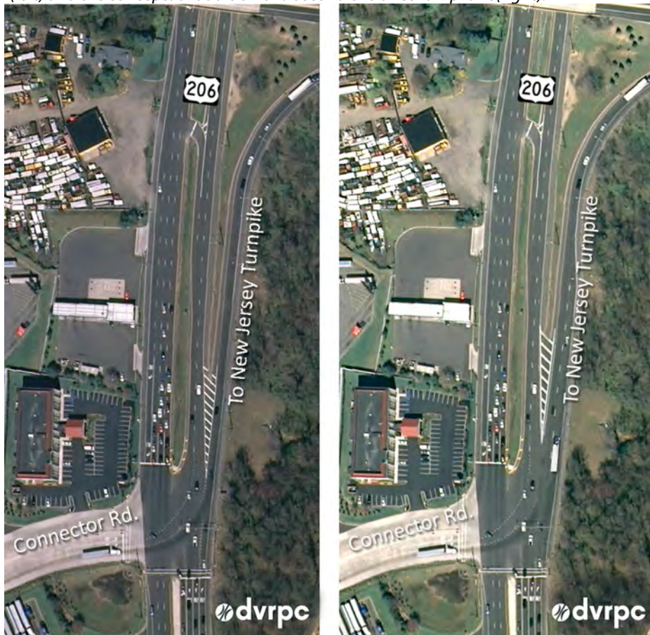
Figure 6: US 206 and Connector Road/NJ Turnpike Entrance - the existing condition (left) and the conceptual addition of a second entrance ramp lane (right).
