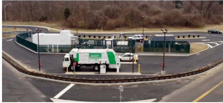
Figure 24. Hauppauge fast-fill compressed natural gas station
