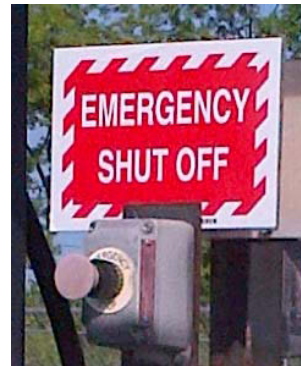
Figure 12. Emergency shut-off buttons for compressed natural gas maintenance facilities and fueling infrastructure
