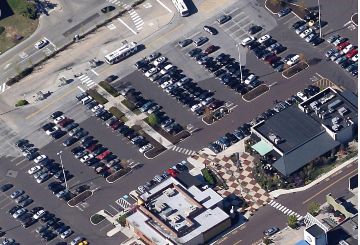
Figure 9: Pedestrian Walkway at Plymouth Meeting Mall Transit Center
