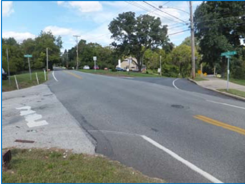
Northbound view of Eagleville Road approach. Source: DVRPC, 2014.
