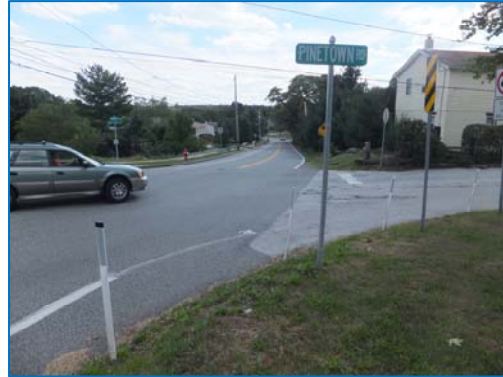
Southbound view of Eagleville Road approach. Source: DVRPC, 2014.
