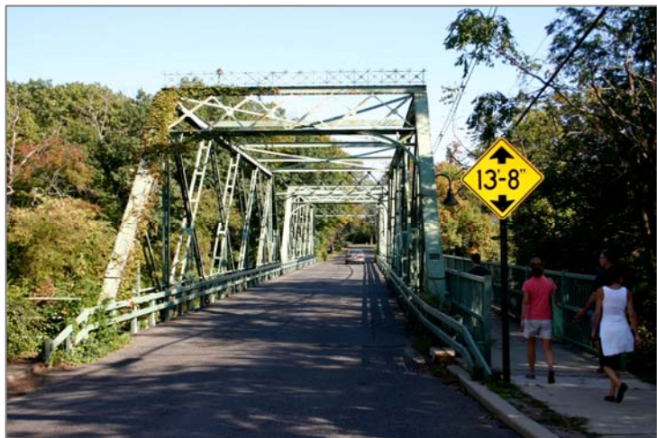
East Ward Avenue Bridge
