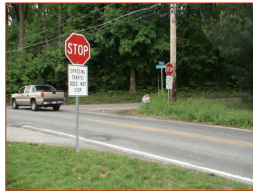
View of Charlestown Road southbound approach. Source: DVRPC, 2012.
