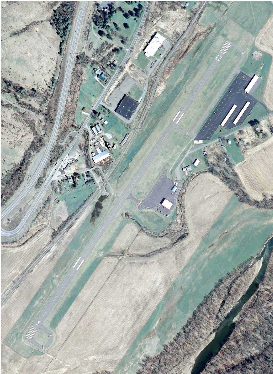
Figure 6: Bradford County Airport (N27) Aerial Photo
