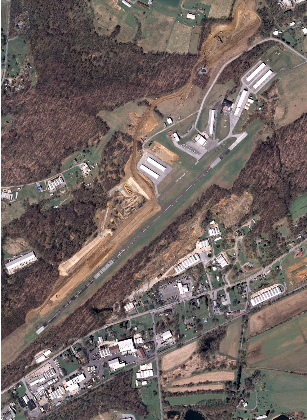
Figure 14: New Garden Airport (N57) Aerial Photo
