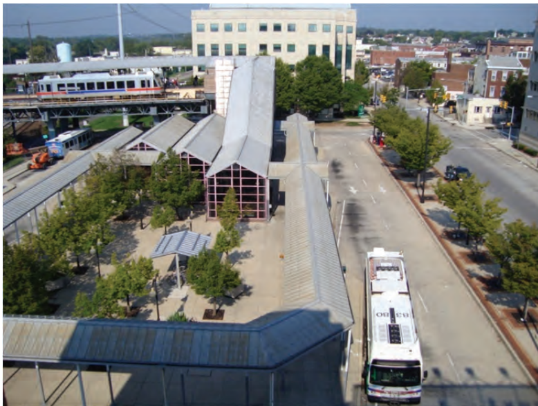
Sawtooth open bus bays at Norristown Transportation Center (Source: DVRPC 2011)
