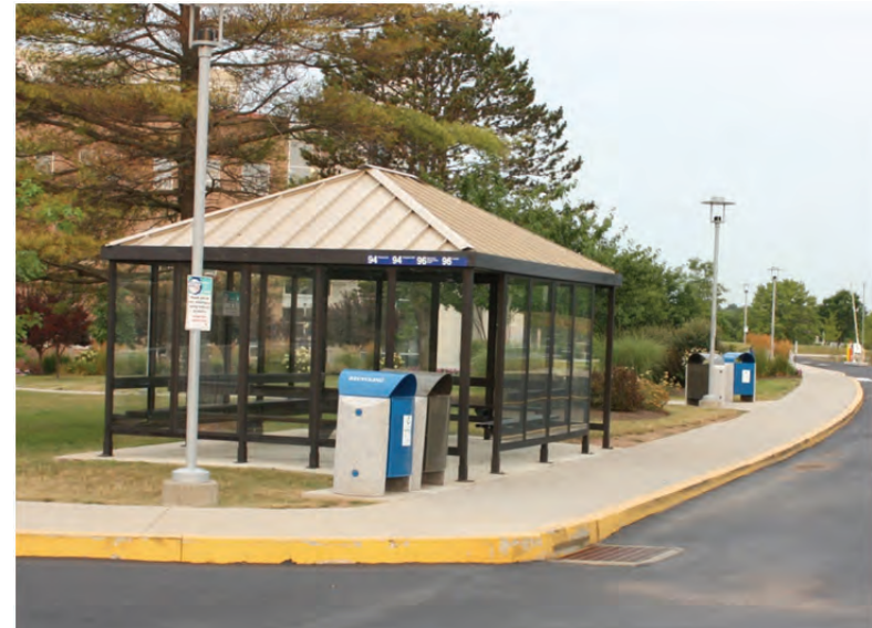
Large shelters such as this one at Montgomery County Community College can accommodate higher numbers of waiting passengers (Source: SEPTA 2012)
