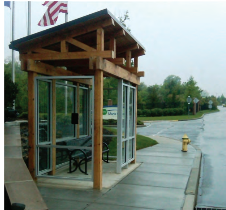
Custom shelter serving retirement community, Glen Mills, PA (Source: SEPTA 2012)
