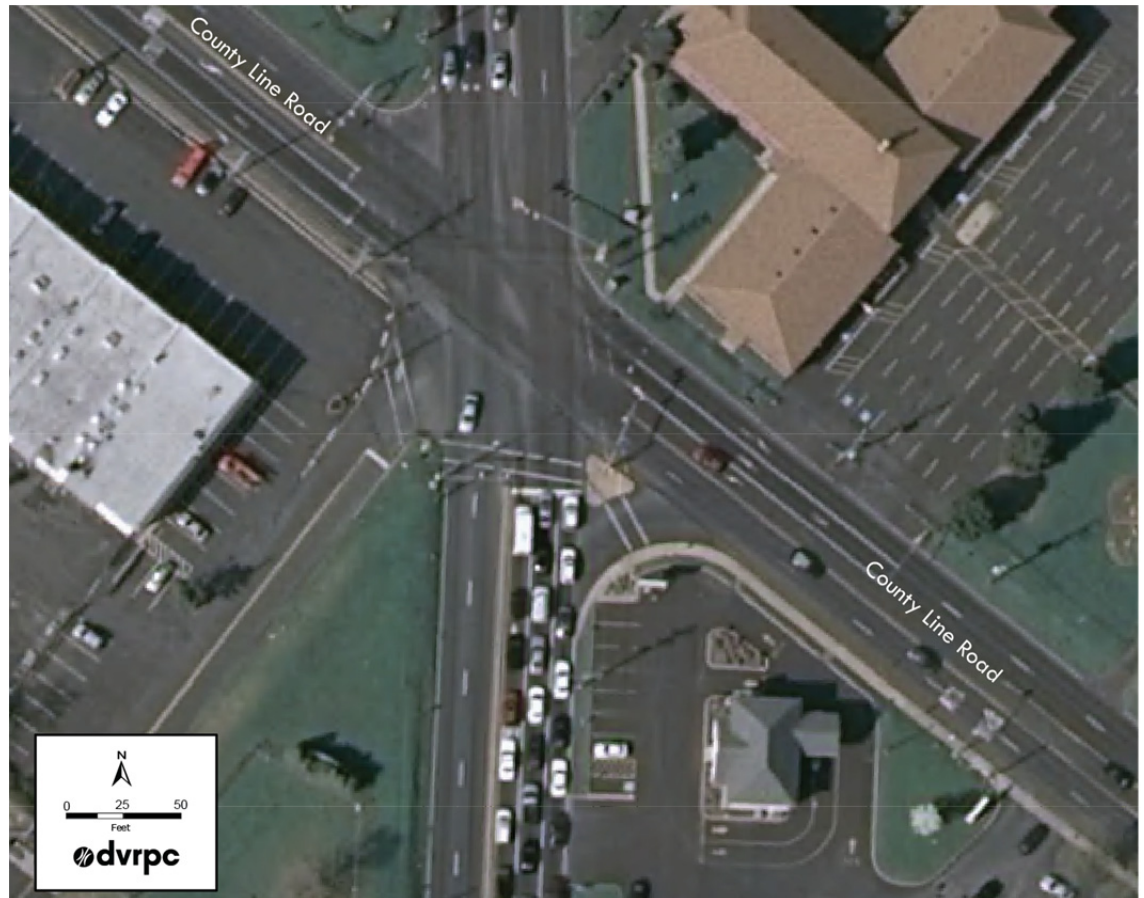
Figure B-1: County Line Road Existing Conditions
