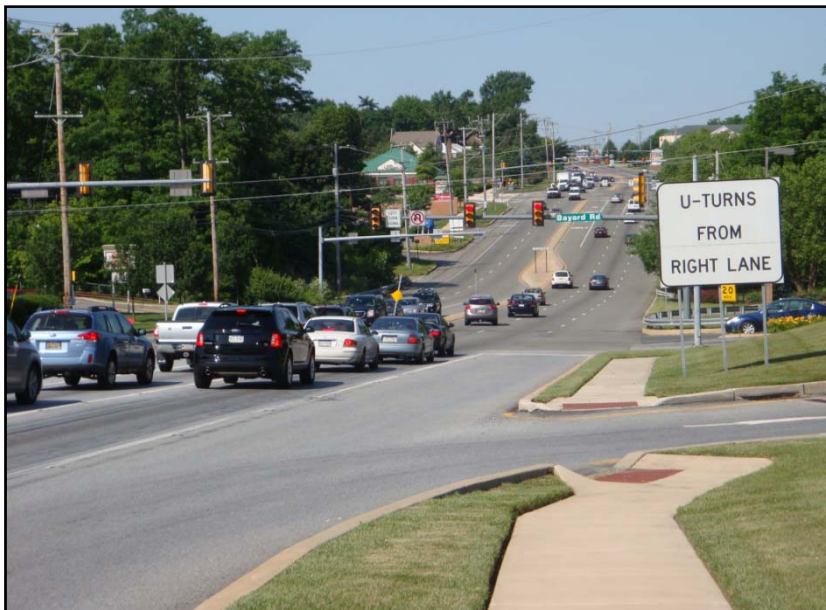
Figure 10: US 1 Five-Lane Configuration
