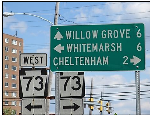
Standard 3-line destination / directional sign—PennDOT D- Series signs—northbound PA 611 at the PA 73 intersection (DVRPC)
