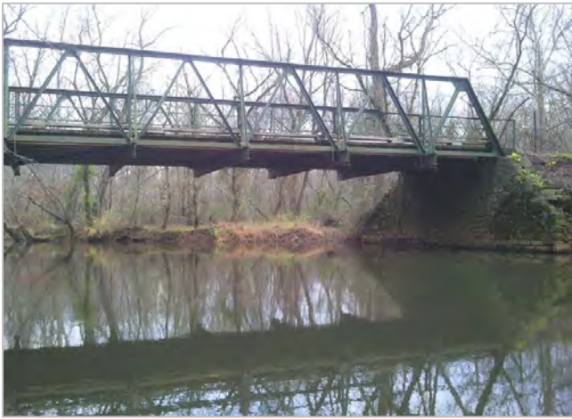
Iron Bridge Road Bridge
