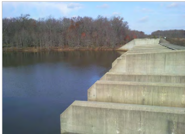
The dam at Van Nest Refuge
