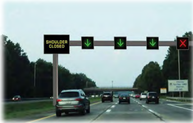
Active Traffic Management allows for shoulder to be closed outside of peak travel periods.
