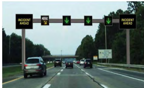
Active Traffic Management allows for travel lanes on I-476 to be closed nearly instantaneously. Photo Source: Virginia Department of Transportation
