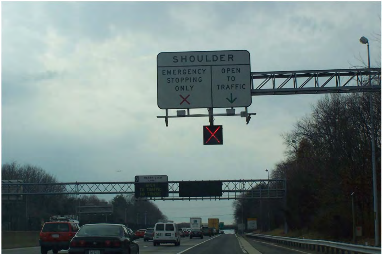
Examples of short-term and mid-term solutions: static and dynamic signing for hard shoulder running Photo Source: RK&K
