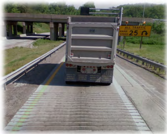
A combination of transverse rumble strips, static warning signs, and speed-based active advanced warning signs have proven effective in reducing accidents due to excessive speeds, as shown on I-79 in Washington County, PA
