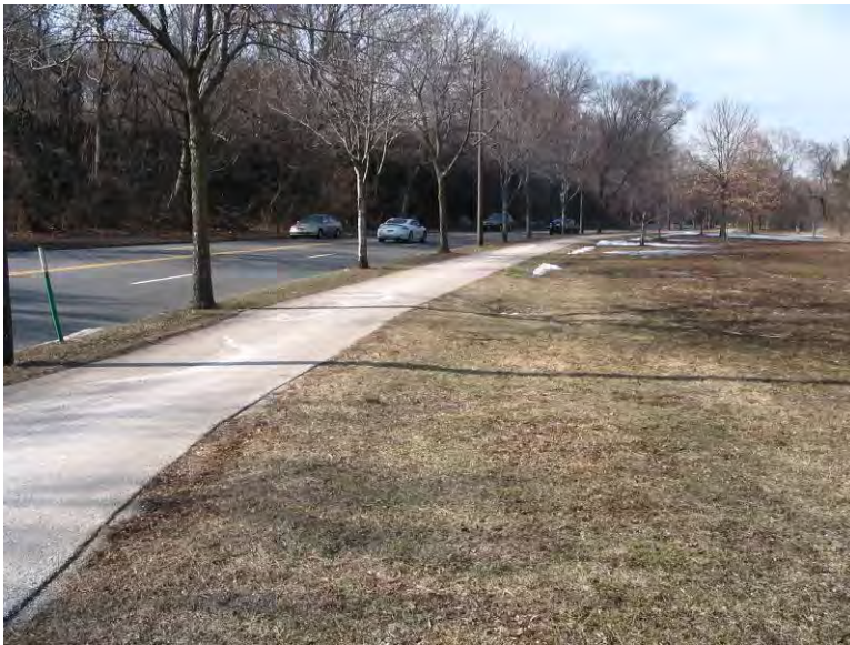
Figure 11: MLK Drive path, just north of Sweetbriar Drive, facing north
