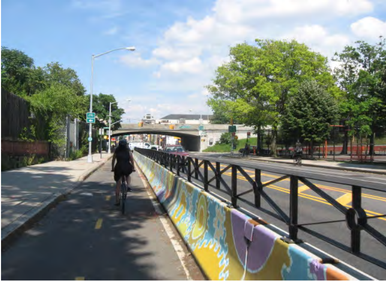
Figure 16: Two-way cycle track in Brooklyn, NY, with enhanced Jersey barrier buffer
