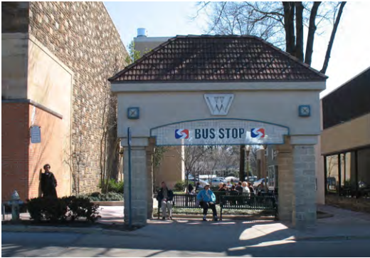
Bus shelter at the Wynnewood Shopping Center.
