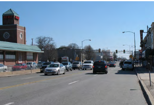
Striping the parking spaces will delineate the travel lanes and encourage drivers to park closer to the curb.
