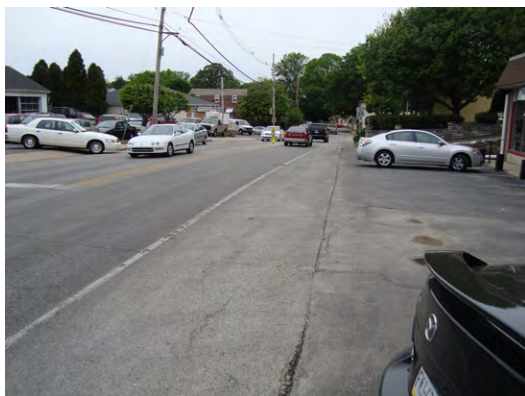
Improving sidewalks, like this one in Garrett Hill, will make Conestoga Road more pedestrian-friendly.
