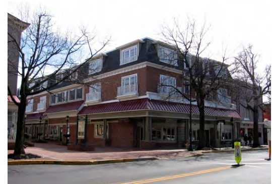
Kings Court in Haddonfield, NJ was designed to complement the scale and context of its surroundings.
