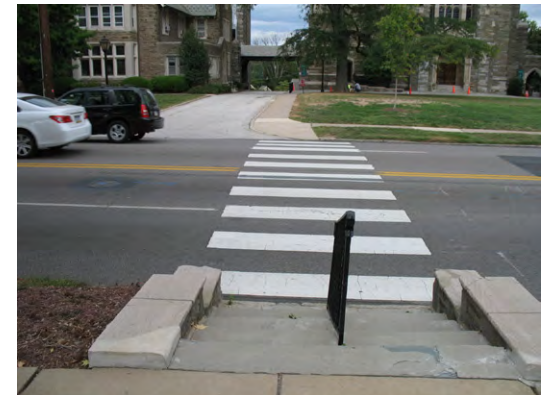
Additional signage and markings can make the this mid-block crossing at Harcum College more visible to drivers.
