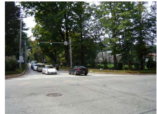
Widening the southern approach to Spring Mill Road would allow right turns to be made while vehicles wait to turn left onto Montgomery Avenue.
