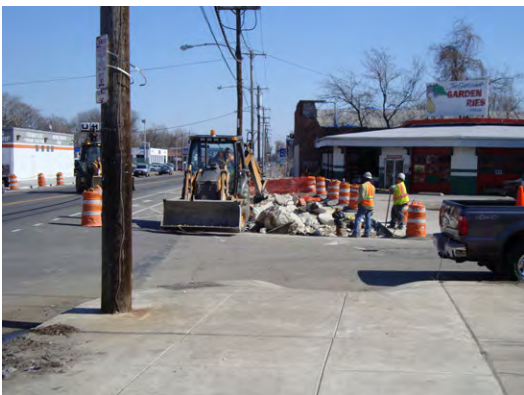
New sidewalks were recently installed in portions of Sub-area 1.
