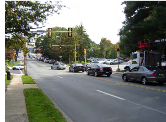
A lead left-turn phase will enable eastbound drivers to more easily make the turn at Airdale Road.
