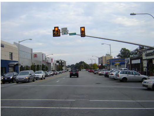
An edgeline is needed to delineate the eastbound traffic lanes.
