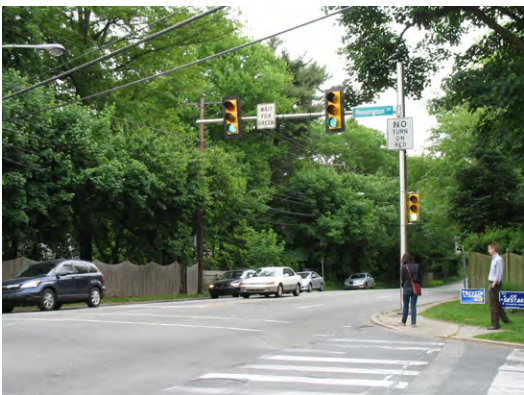
Curb ramps and pedestrian countdown signals are needed at the intersection of Lancaster Avenue and Remington Road.
