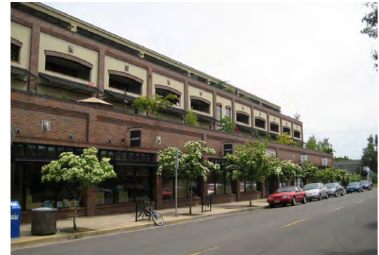
This four story building utilizes step backs to minimize its overall height.
