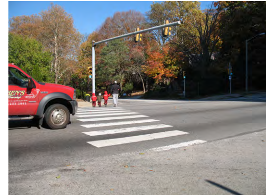
Pedestrians crossing City Avenue at Drexel Road.
