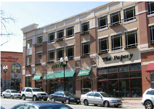
This mixed-use garage in Arlington, VA does a good job of blending into the neighborhood.
