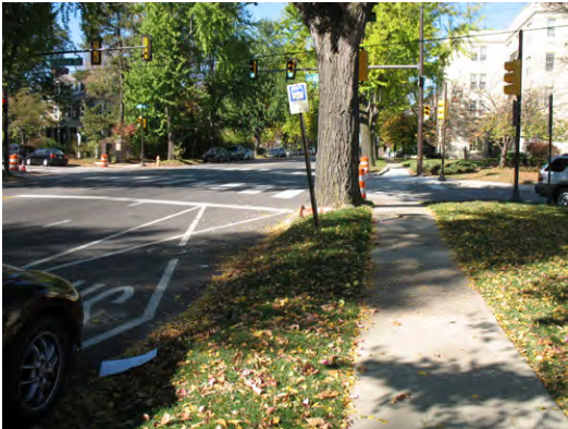
Pedestrian countdown signals were not installed at the intersection of Lancaster Avenue and Overbrook Avenue.
