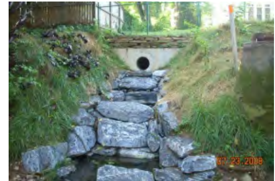
Step pools outlet retrofit. Photo: Montgomery County, Maryland DEP
