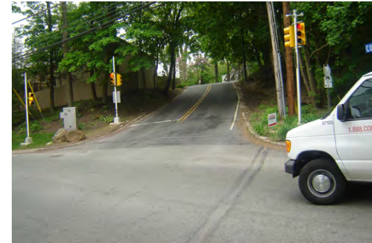
Installing mast arms at Radnor Chester Road can help improve the visibility of traffic signals.
