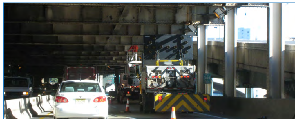
I-76's westbound lanes, adjacent to Center City, are built on pilings which also support the "30 th Street deck." Eventual replacement is a concern to PennDOT. (DVRPC)
