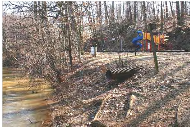
An Exposed Outfall at Lake Narraticon Park
