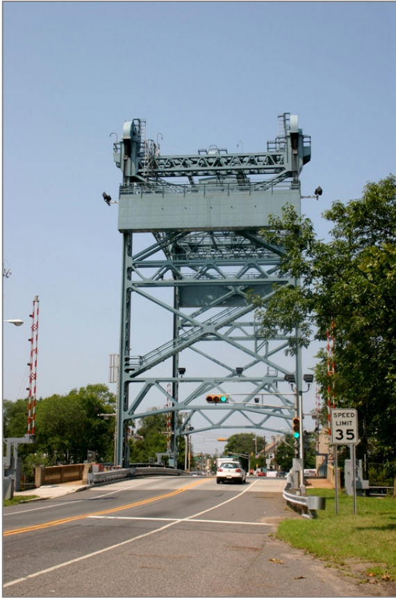
NJ Route 44 Mantua Creek Bridge
