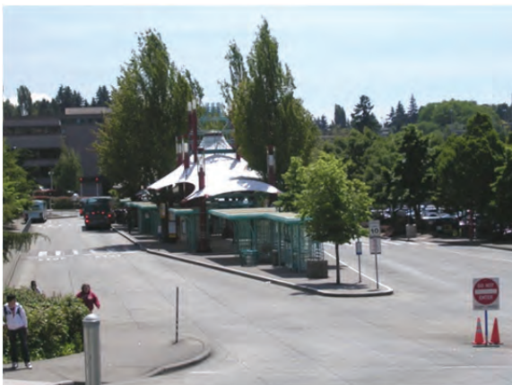
High-quality bus transfer hub at shopping mall near Seattle, WA ( Source : DVRPC 2010)
