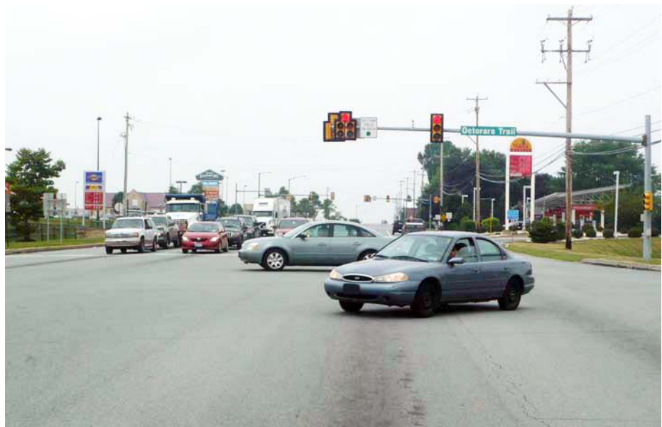
High traffic volumes, high speeds, and many possible movements contribute to the US 30 and PA 10 intersection being the most crash prone in the corridor. DVRPC, 2009
