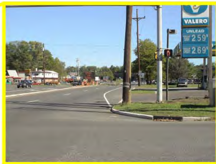
Missing pedestrian crossings and curb ramps on select approaches of the Farnsworth Avenue and US 130 intersection
