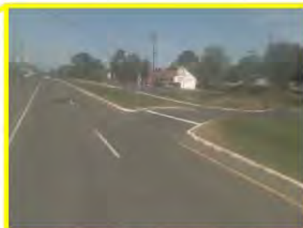
Limited sight distance on US 130 SB ramp cross-over
