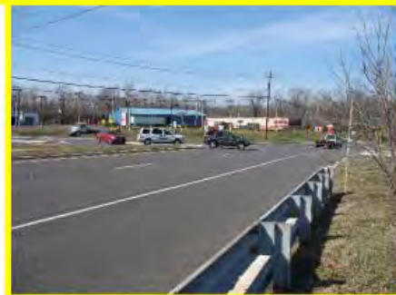
Limited sight distance and high travel speeds occur where there is cross-over access from the access road to 206 NB and Mastori's Restaurant
