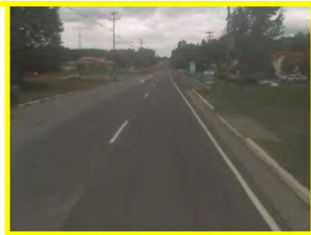
No advance warning of traffic entering US 130 NB from cross-over
