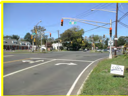
Missing pedestrian crossing accommodations on every leg of intersection
