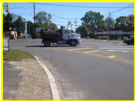
Dedicated right turn lane at Crosswicks intersection creates unsafe conditions for pedestrians and bicyclists
