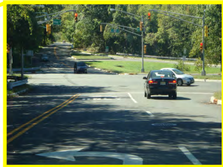
No pedestrian accommodations at intersection
