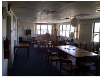
Photo 2 – Pilot's lounge and kitchen
