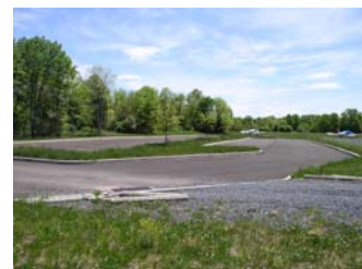
Photo 6 – North Hangar Car Parking
