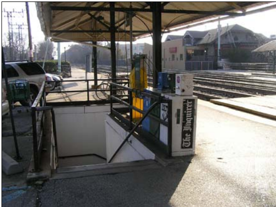
An underground passageway allows transfer between both sides of the station.
