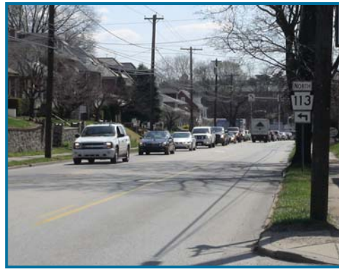
Residences along the north side of Nutt Road (Source: DVRPC)
