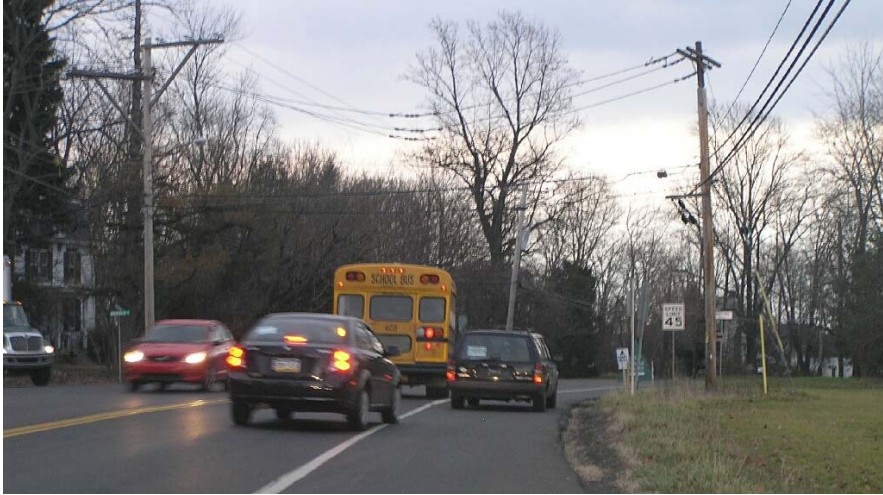
Durham Road southbound approaching Stoopville Road: Wide shoulder allows through traffic to bypass stopped left turning vehicles (the school bus in the photo). Photo by: DVRPC
