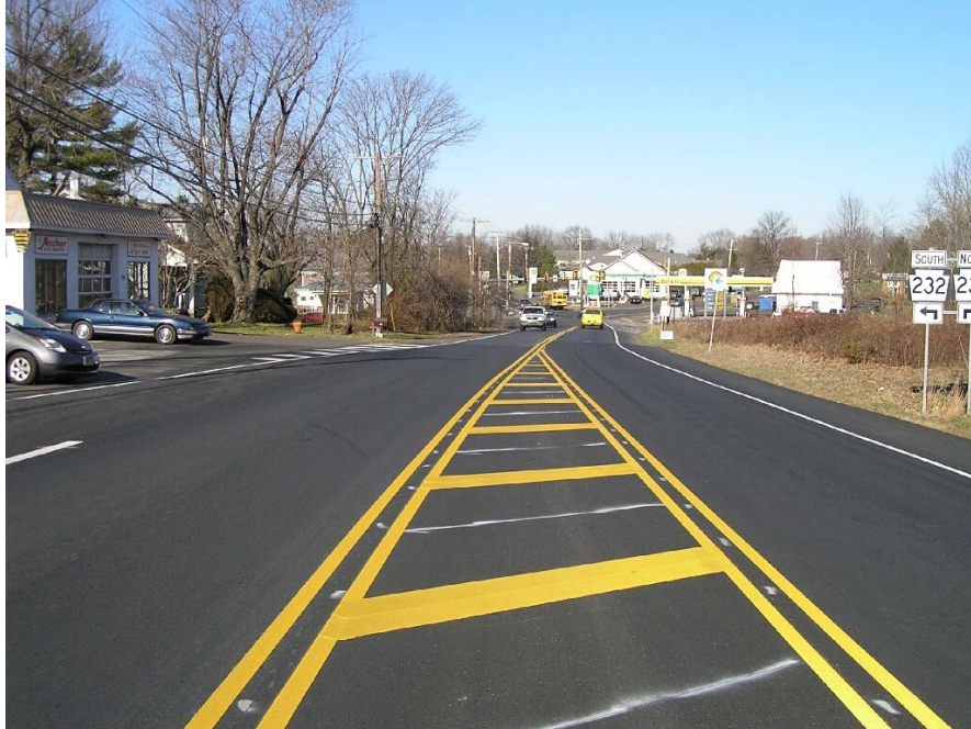
Durham Road northbound, near Anchor Road: The automotive repair shop (on the left) has "open" access to PA 413 along its entire frontage. Photo by DVRPC
